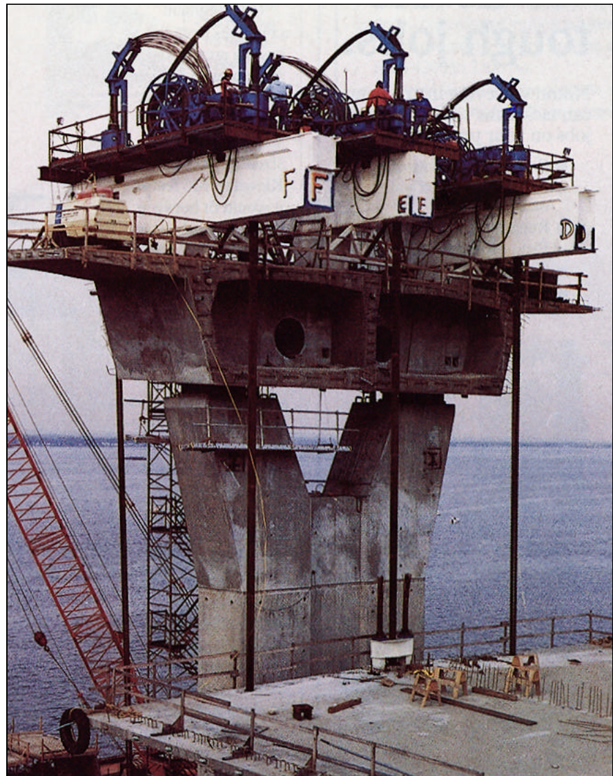
Six 1,000-ton jacks mounted on steel box beams atop the pier segment of the bridge provide lifting power at each end of the 2,400-ton precast girder.
